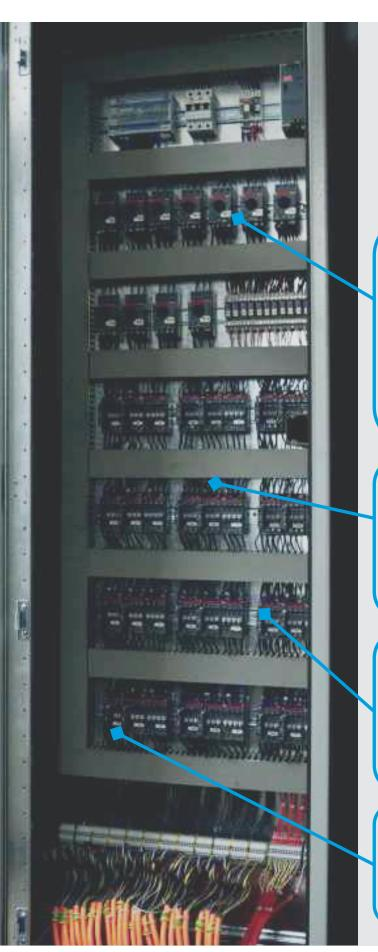
Automation panel is responsible for operating in accordance with the ventilation scenarios processed. PLC (Programmable Logic Card) which is carried by all mechanical devices (axial fans, jet fans, air / smoke dampers, doors etc.) in the system according to the signals coming from the carbon monoxide detection system and / or fire / smoke detection system which analyzes the situation in the parking lot.
